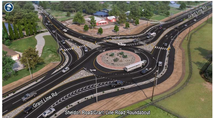
Segment C – Grant Line Road Roundabout
