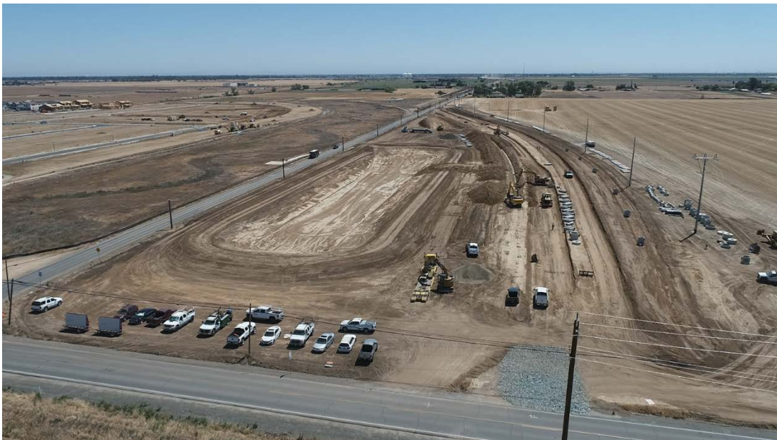
Picture 1 – Detention basin roadway grading near Bruceville Rd
