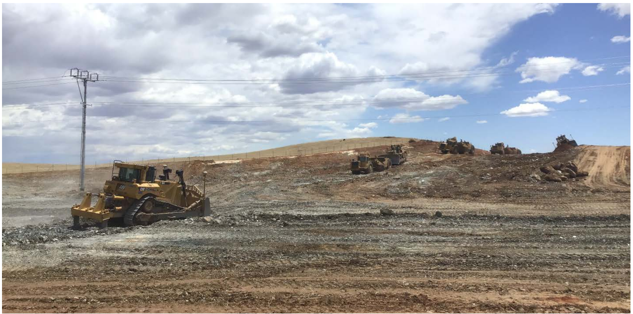
Picture 5 – Roadway Excavation
