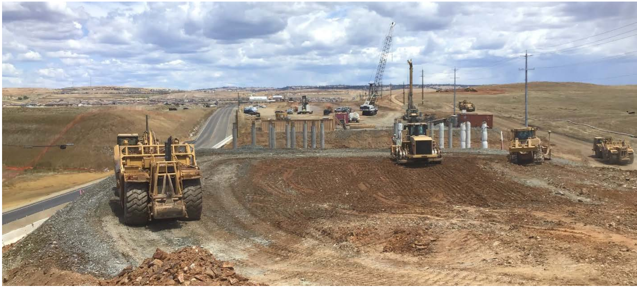
Picture 4 – Bridge foundation construction at Alder Creek
